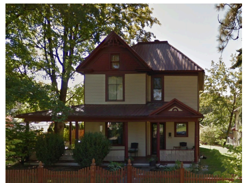
Figure 34. 712 E Foster Avenue
